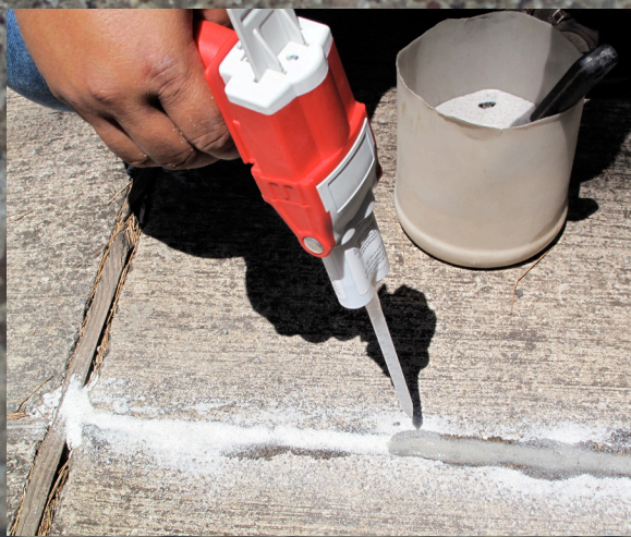
Repair walkways and patios.
